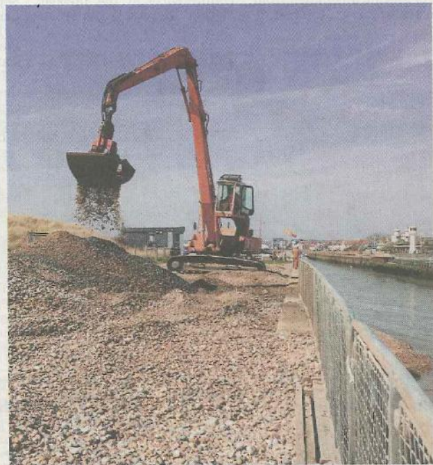
The excavator removing shingle from the harbour
